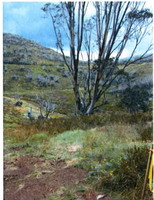
Photograph 2: Tree to be removed. Stake to the right is the start of the lateral trench.
